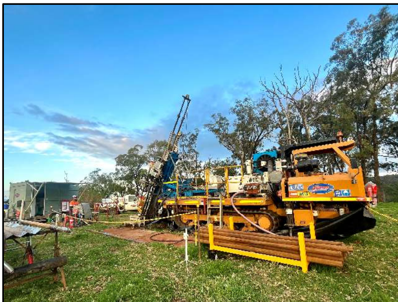
Figure 1 – May Queen – Drilling in progress at MQDD002
